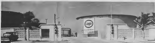
Lago's Main Gate has a new appearance after a refinery fence beautification program.
